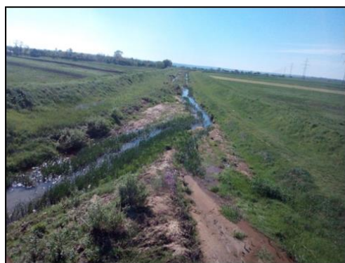
Fig. 5 The dam of the Drincea river - Punghina settlement (April 2017)
