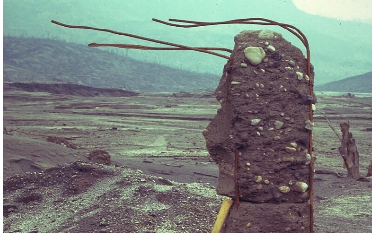
Fig. no 6. Burning volcanic clouds are a mixture of volcanic gases and tephra. Their destructive effect is determined by high temperature that leads to fires, and by high pressure due to considerable thickness of clouds and high speed of their displacement. This photo shows the ruins of a house in the village of Francisco Leon destroyed by the burning volcanic cloud during the El Chichon volcano eruption, South-Eastern Mexico from March 29 to April 4, 1982. The reinforcing concrete bars in the ferroconcrete wall are bended in the direction of the burning cloud movement. Several clouds of this kind moved in different directions from the volcano from 2 to 8 km. Besides the village of Francisco Leon situated 5 km from the volcano, 8 more villages were destroyed. More than 2,000 persons. Photo Credit: R. I. Tilling, June 1, 1982
