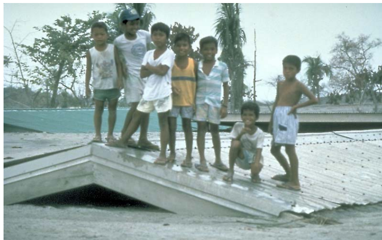
Fig. no 7. Volcanic mudflows (lahars) appear when the water-sodden ash glides down volcanic slopes. The photo shows the lahar-buried school after the eruption Pinatubo volcano, Philippines which started in June 15, 1991. As thousands other buildings this school was damaged. Photo Credit: T. Pierson, October 12, 1991
